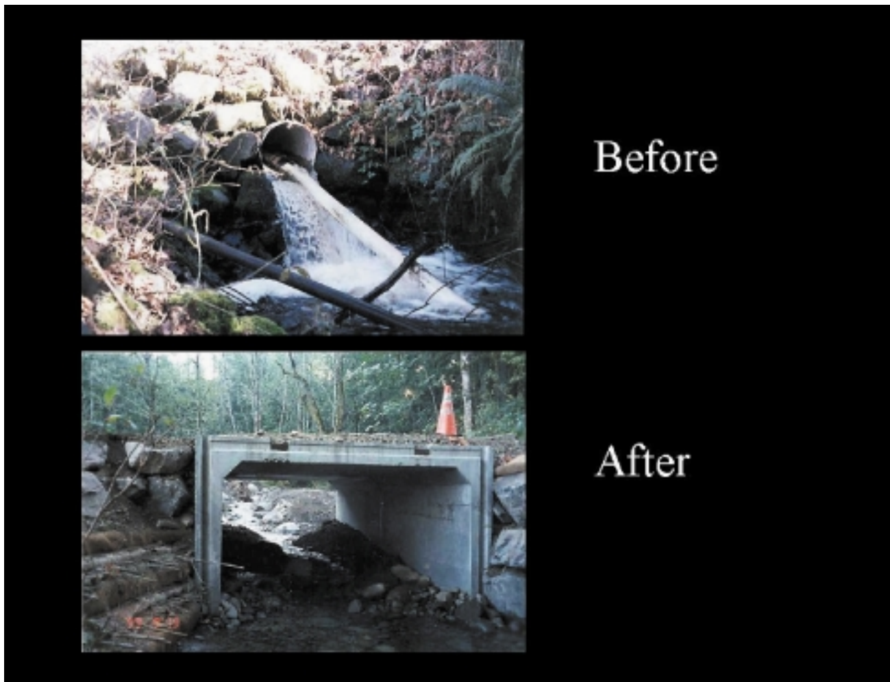
Figure 8. Culvert replacement for fish passage at O'Grady Creek (Photos taken immediately before and after construction)
