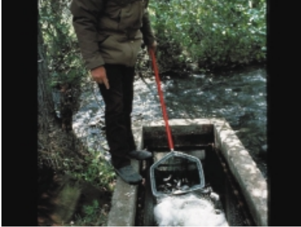
Figure 14. Screen bypass trap box (fish saved by screen are sorted by species and counted; steelhead smolts in box in photo; John Day River Basin, eastern Oregon)
