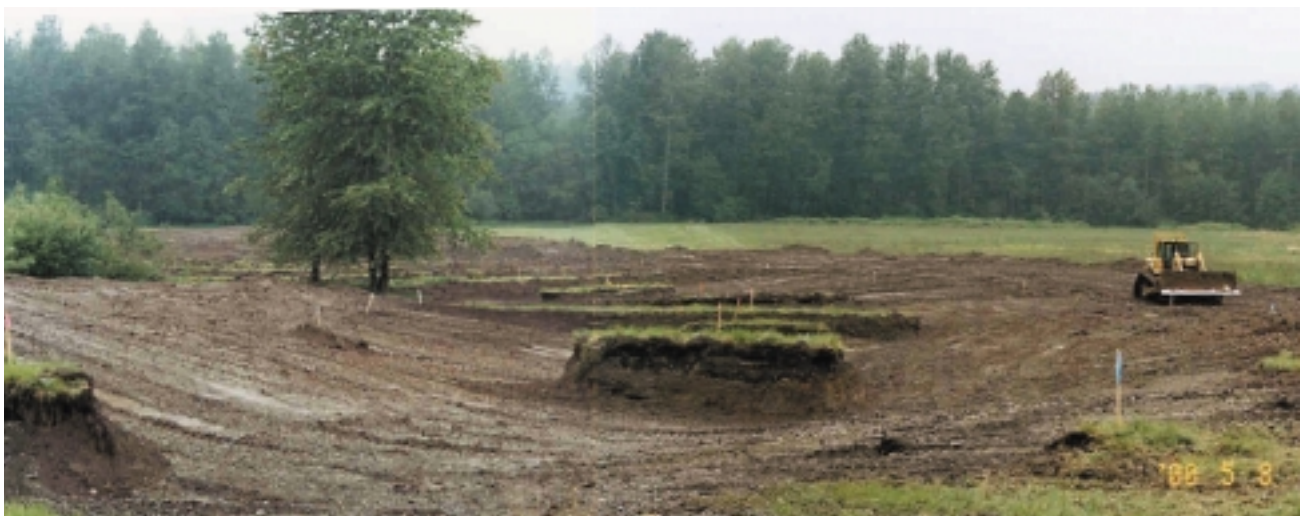
Figure 11. Earthwork to create new stream alignment with floodplain bench, May 2000. Wetland area is to the left side of the photo, and the side channel of the Green River is behind the trees in the background.
