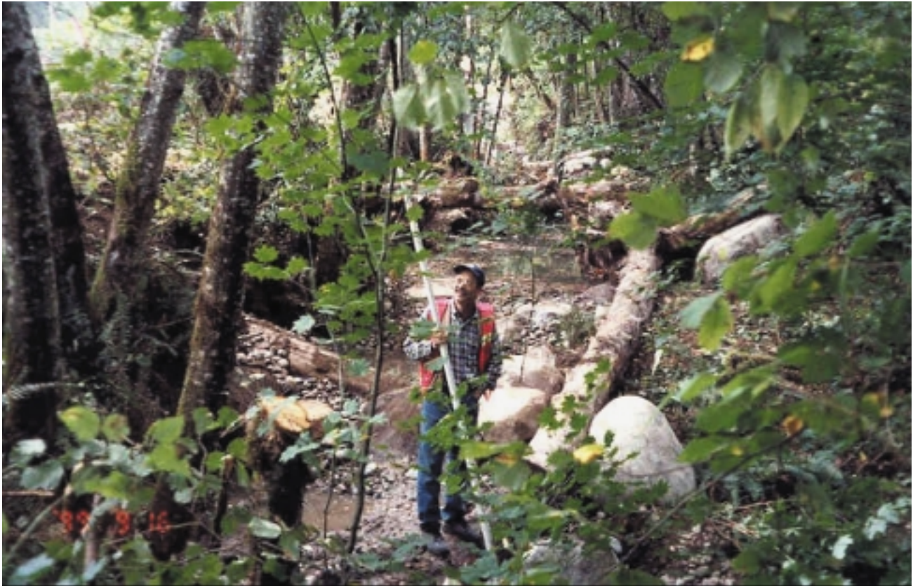
Figure 1. Streambed rehabilitation project under construction. Project design team ecologist checking invert of instream boulder wedge. (Case study project 4)
