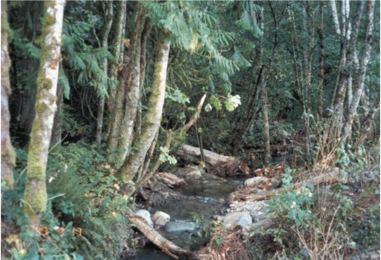
Figure 9. Looking downstream from the new culvert at the rebuilt reach of O'Grady Creek after construction. The streambed here is about three feet higher than the eroded streambed. Buried boulder wedges create a stepped reach of pools for fish passage. LWD was added for habitat diversity.
