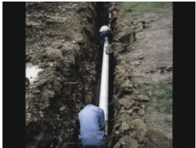
Figure 13. Fish screen bypass (bypass safely returns screened fish to stream; bypass can be very long, even hundreds of feet; eastern Oregon)
