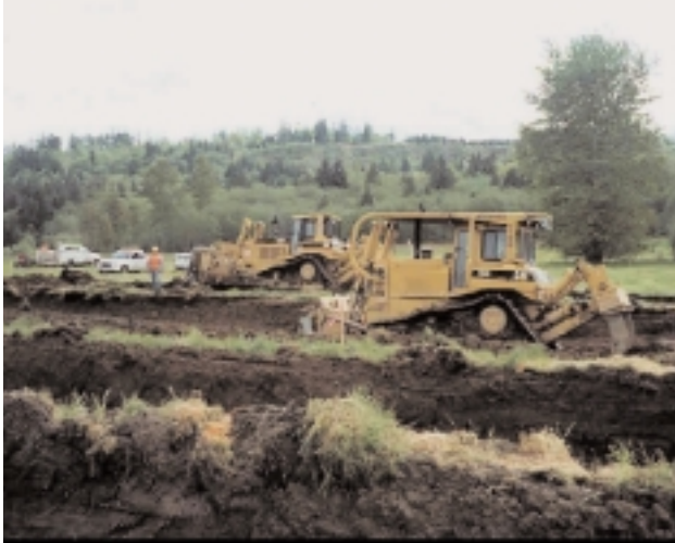
Figure 2. Excavation of defined floodplain for O'Grady creek (Case study project 5)
