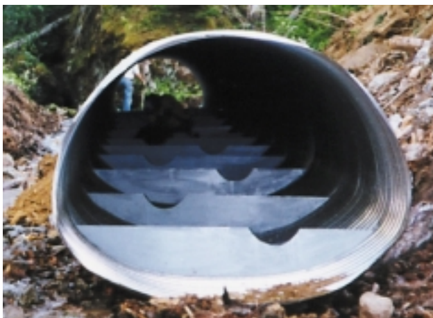
Figure 4. Baffles welded into a culvert
