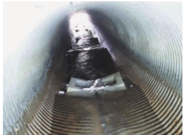
Figure 3. Correctly installed chimney block fish ladder
