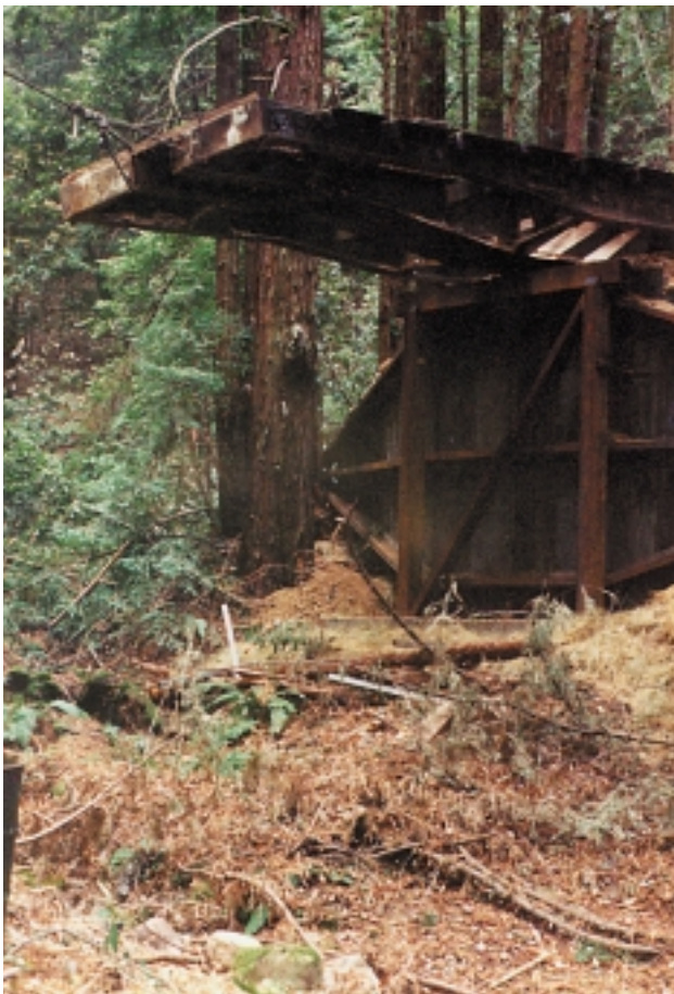
Figure 13. Example of bridge installation bulkheading
