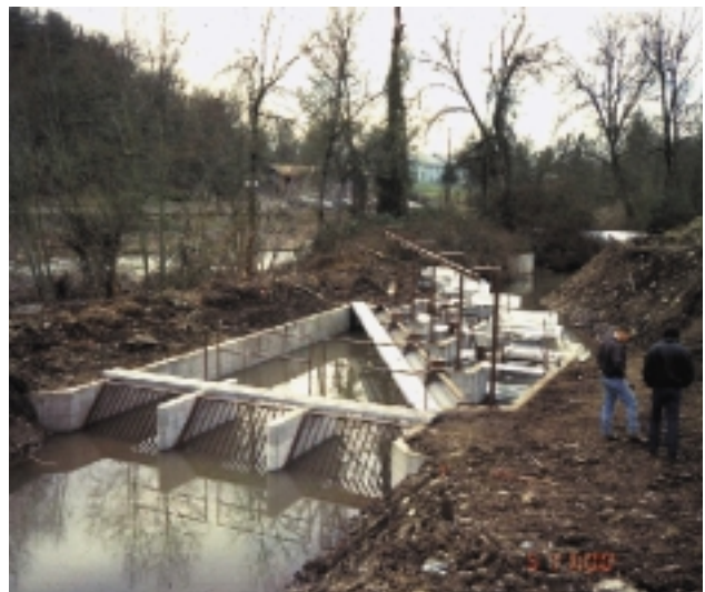
Figure 4. Rotary drum screen (self-cleaning drum screen; paddle powered; four-bay; Rogue River Basin, southwestern Oregon; 29 cfs)
