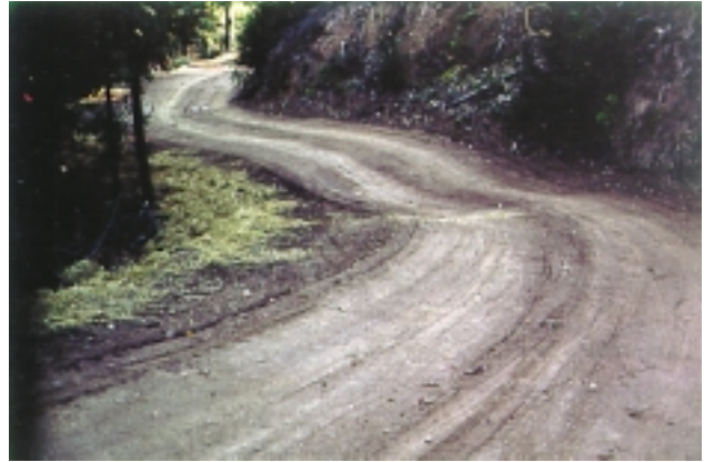
Figure 8. A rolling dip draining surface runoff onto a fillslope covered with strawmulch (Soda Springs Road, Albion River Watershed, CA)
