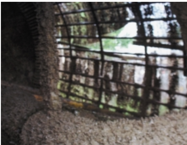
Figure 16. Corroded screen (inside view)
