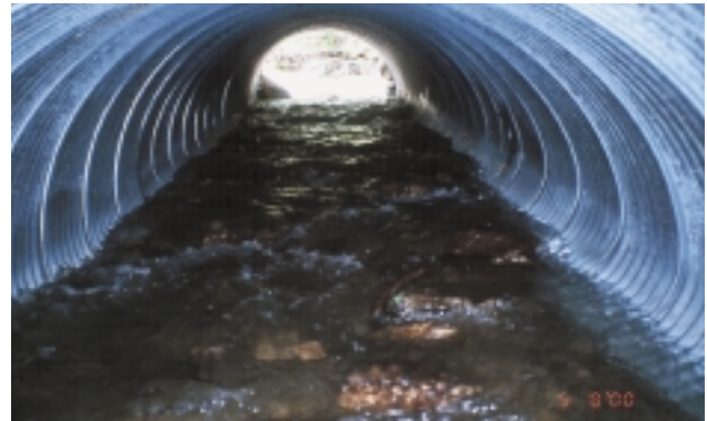
Figure 11. Example of a buried culvert
