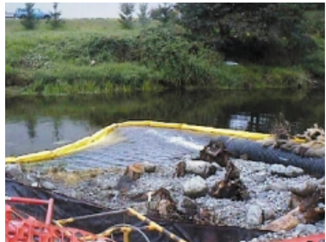
Figure 5. Silt curtain in the Sammamish River
