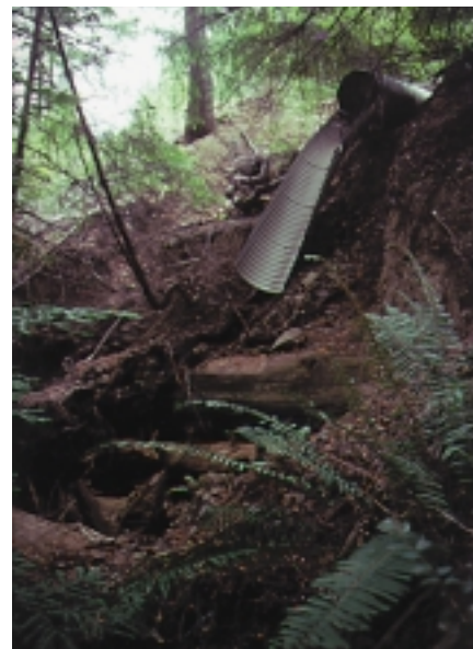
Figure 3. A culvert and downspout installed on top of an old Humboldt crossing (Little North Fork Navarro River, CA)
