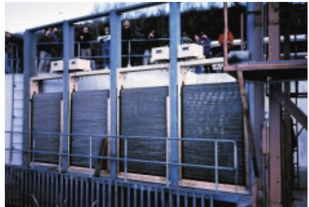
Figure 8. Traveling belt screen (plastic; 10 cfs solar powered screen; eastern Oregon)
