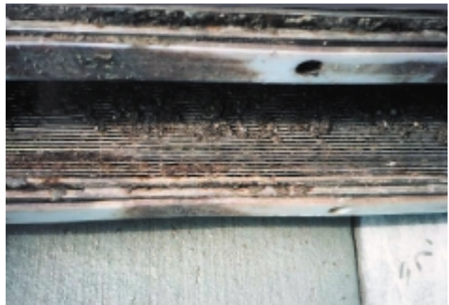
Figure 10. Improperly cleaned and maintained screen
