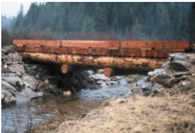
Figure 6. Example of a wood stringer bridge
