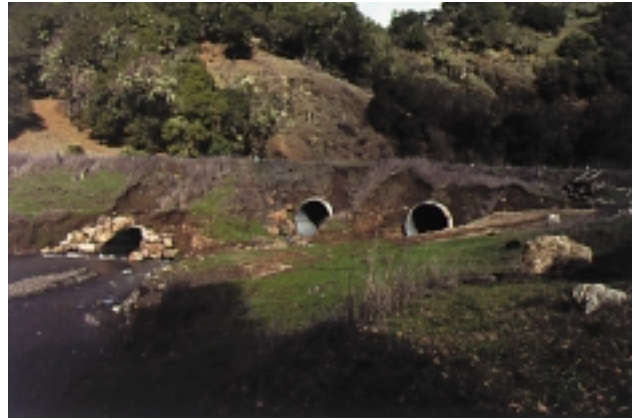
Figure 3. A culvert and downspout installed on top of an old Humboldt crossing (Little North Fork Navarro River, CA)
