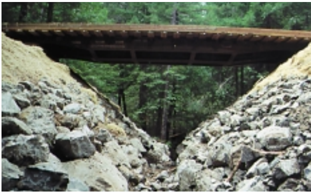
Figure 12. Example of a railroad flatcar bridge installed with riprap along the channel
