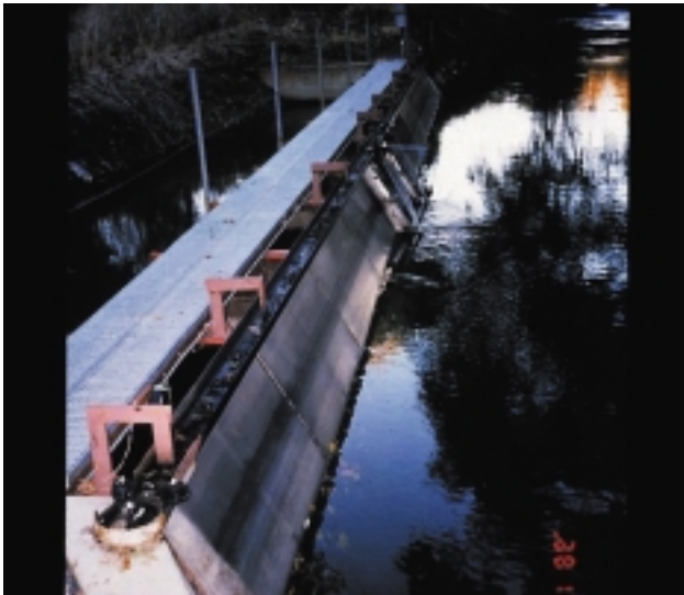
Figure 9. Self-cleaning panel screen (160 cfs wiper brush self-cleaning screen; electric powered; Parrot-Phelan Diversion in northern California)
