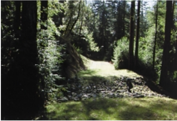
Figure 9. Example of a rock-armored crossing
