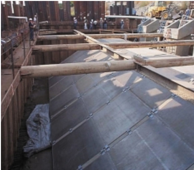
Figure 8. PCG-P's facility behind significant cofferdam
