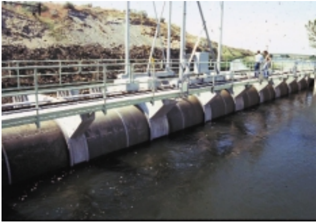
Figure 5. Rotary drum screen (self-cleaning drum screen; electric powered; eastern Washington)
