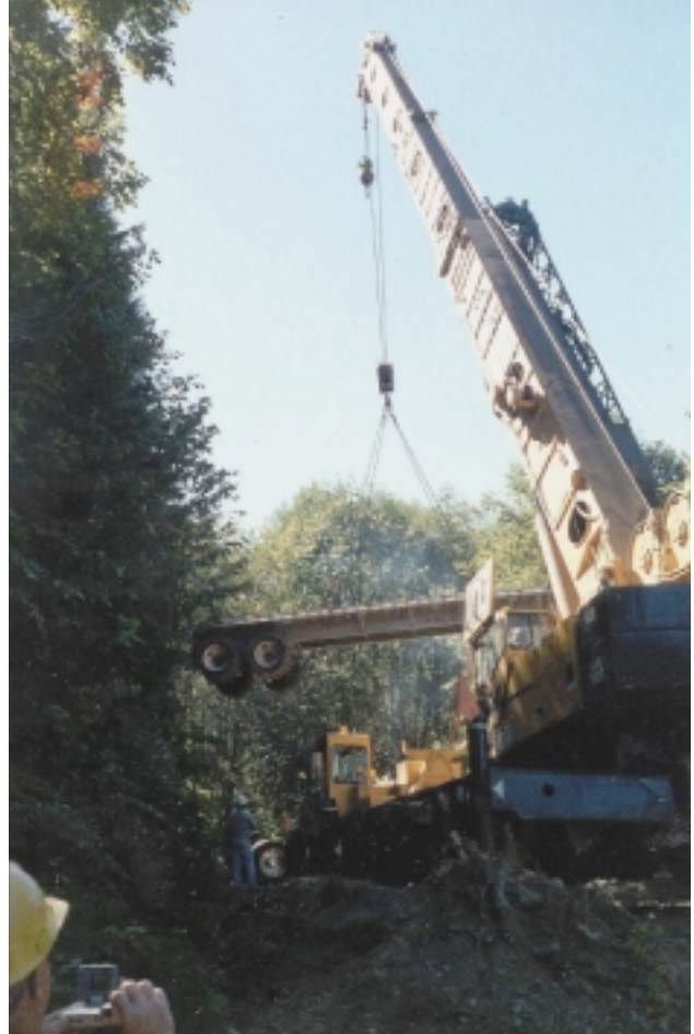
Figure 3. Crane overcomes tight construction access for delivery truck (Case study project 4)
