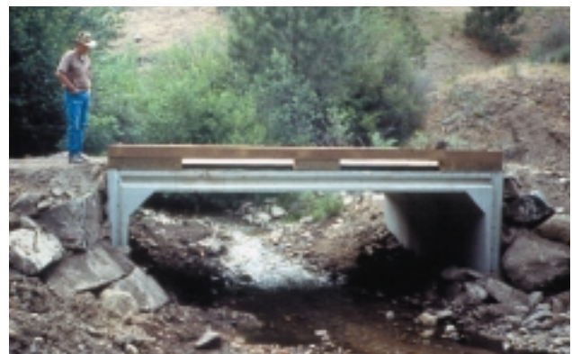
Figure 7. Example of a pre-fabricated concrete bridge
