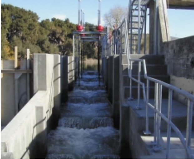
Figure 6. Operational flexibility (adjustable overflow gates allow proper ladder hydraulics with 3-foot pool fluctuation)
